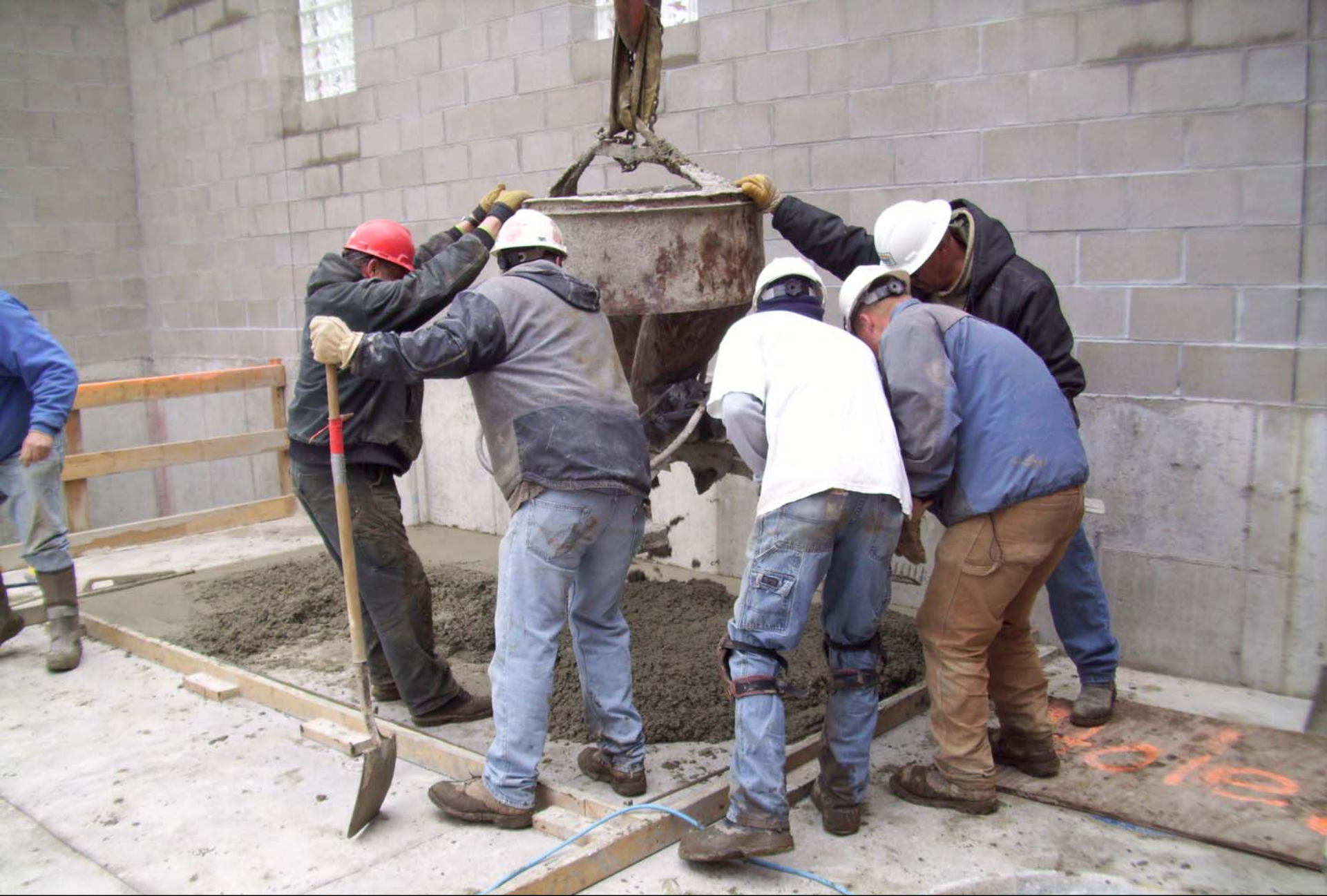
Preparing installation of pads
