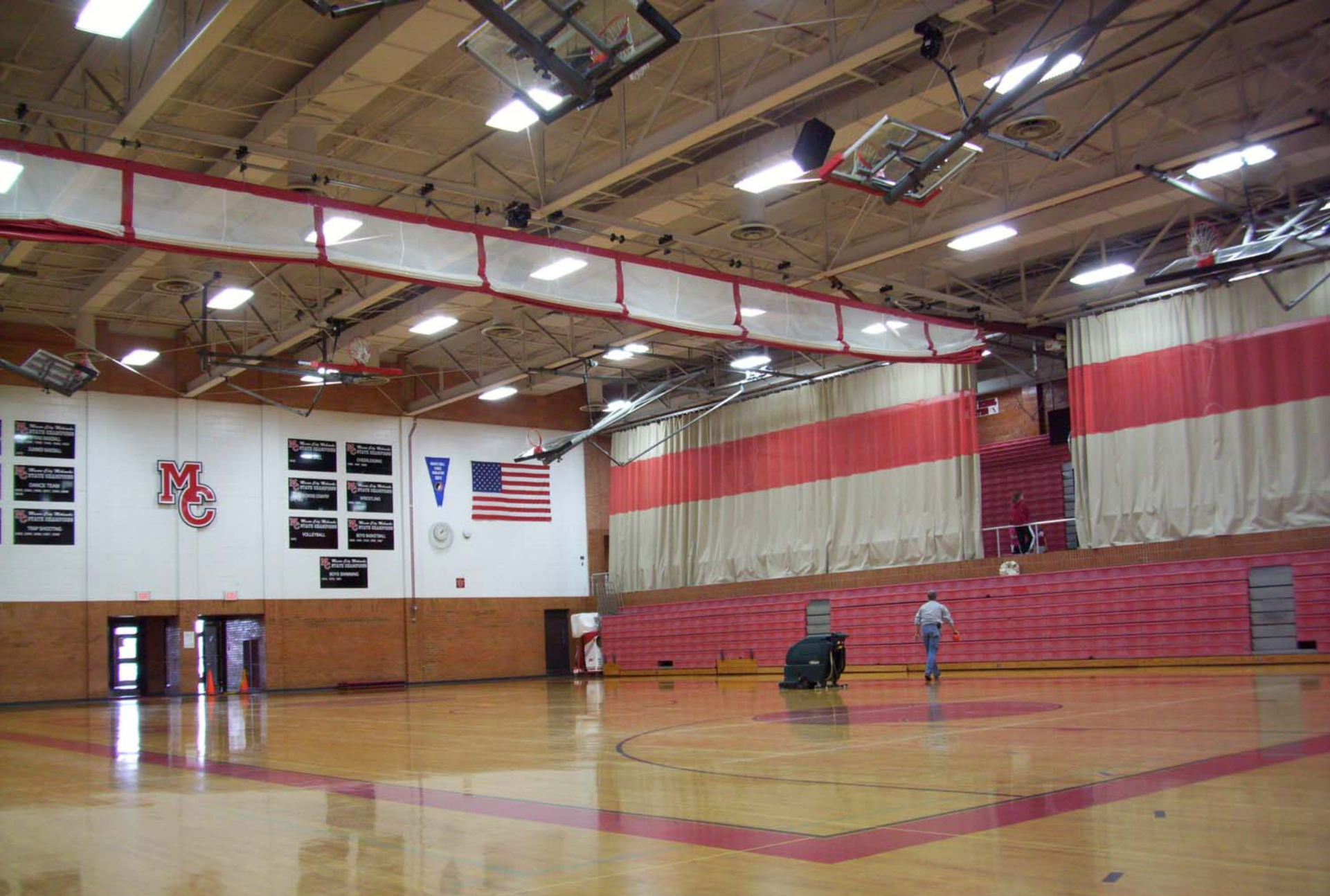
Phase 1 lights for MCHS gymnasium
