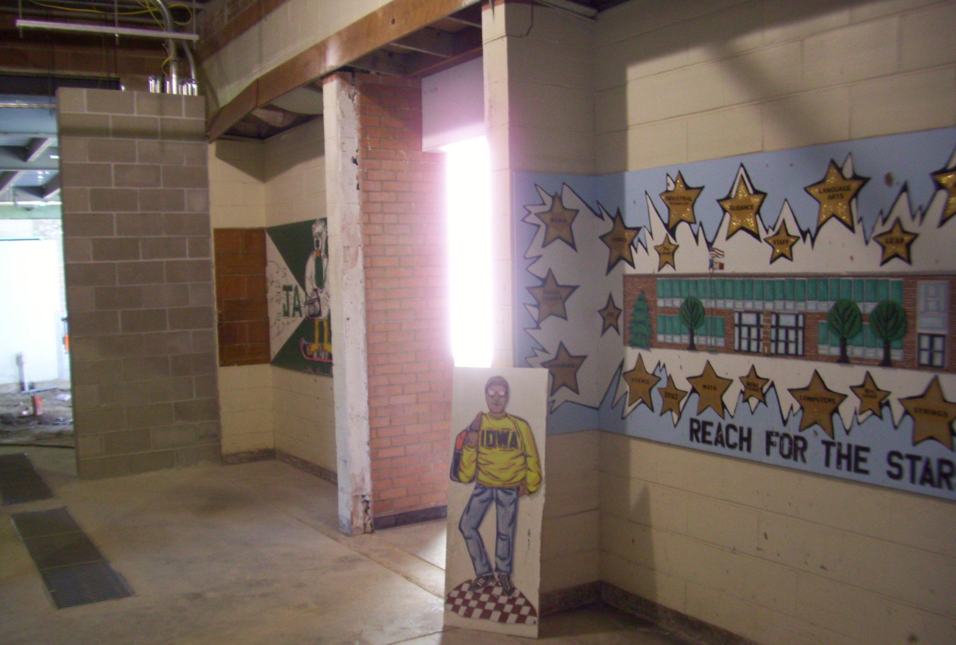
Phase 3A Cafeteria (old cafeteria)
