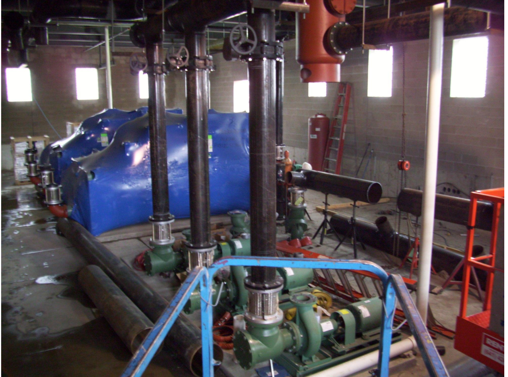
Chiller Water Piping Installation
