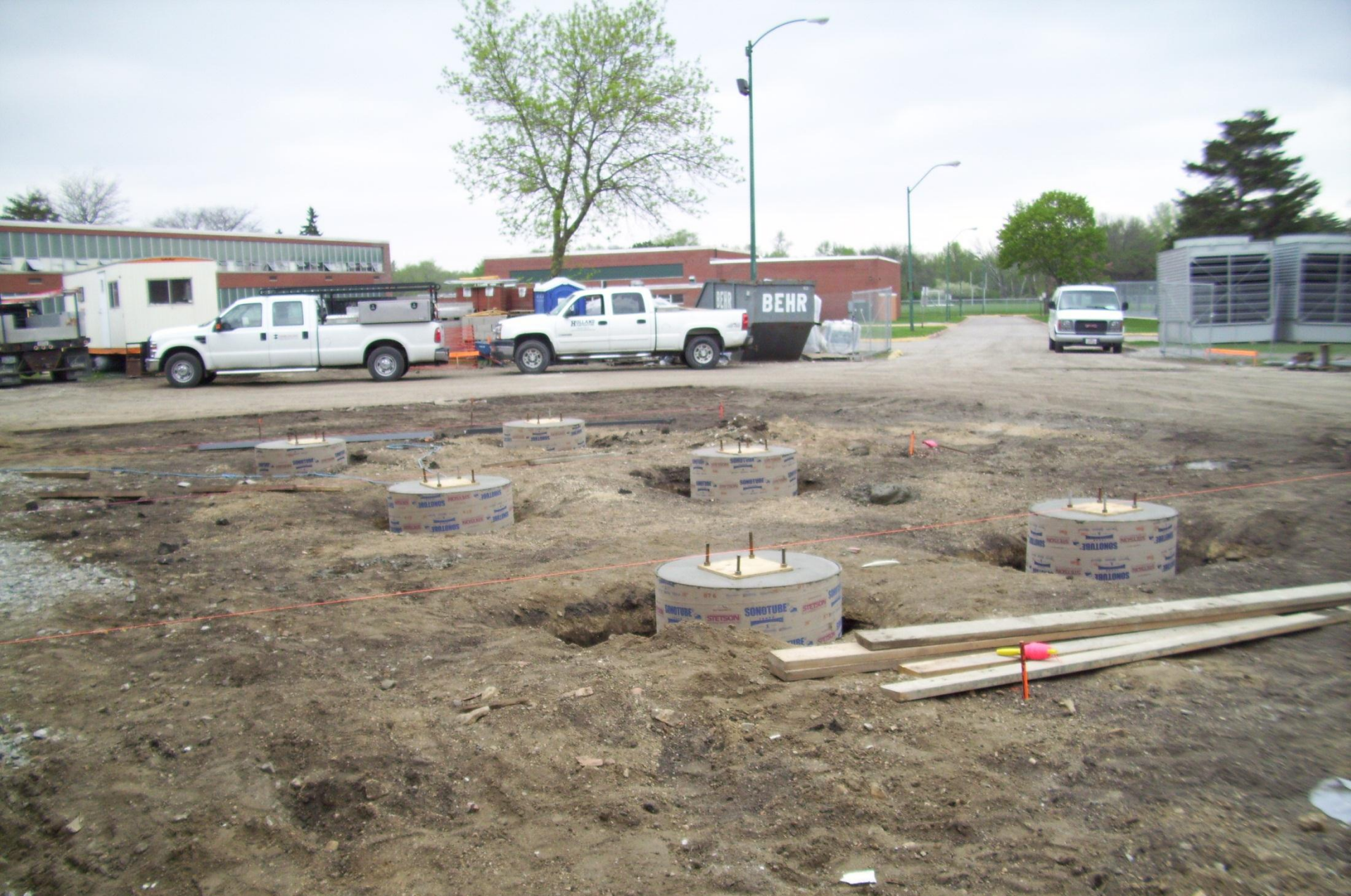
Cooling Tower Footings
