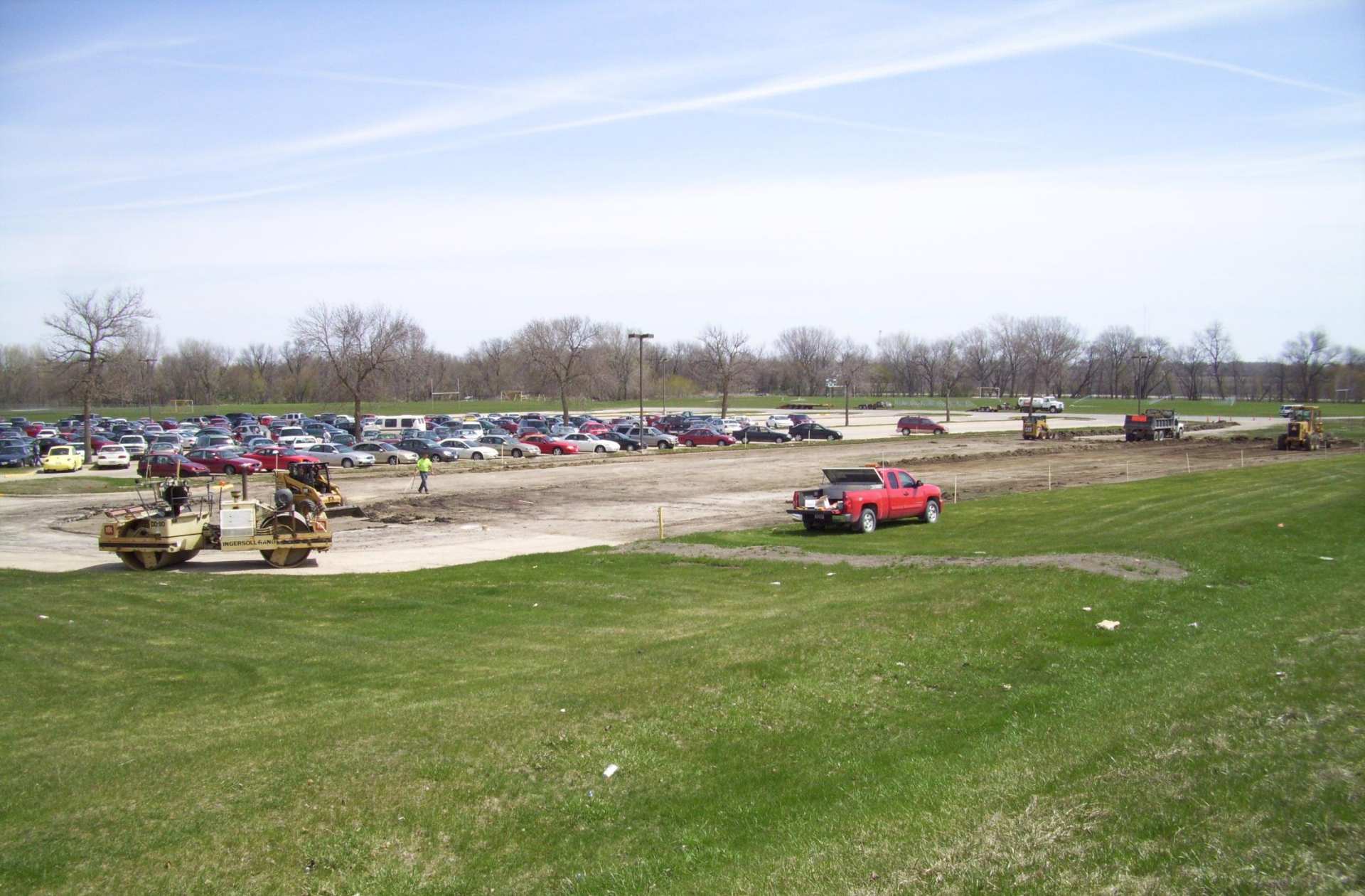
Asphalt Milling Installation of High School Parking Lot
