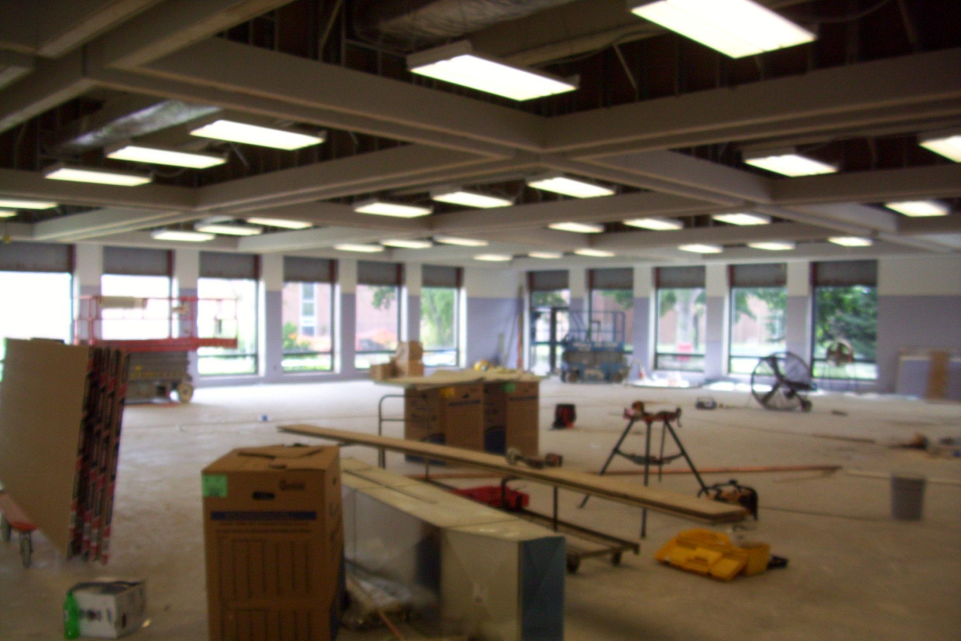
Phase 3A Cafeteria Temp
